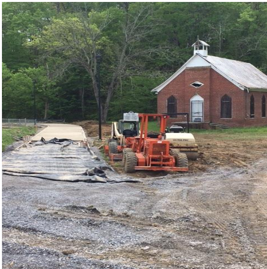
Middle Creek Greenway construction near New Salem Baptist Church.
