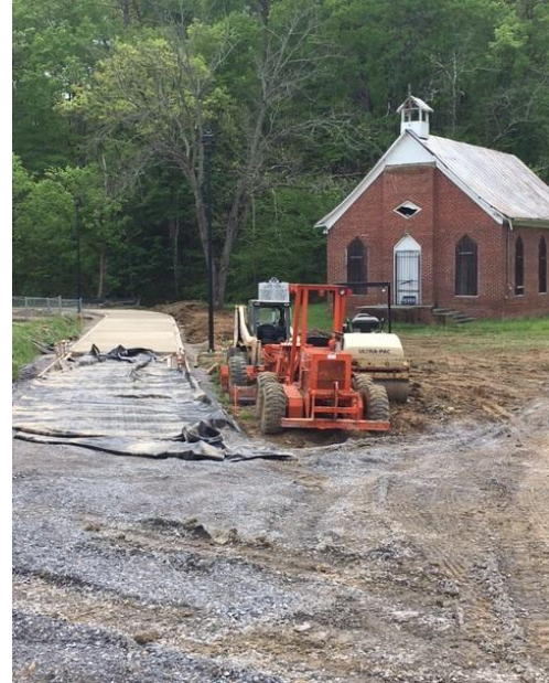
Middle Creek Greenway construction near New Salem Baptist Church
